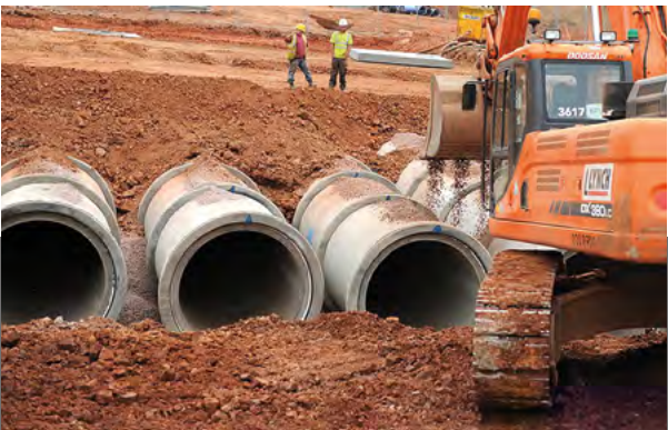
Concrete drainage does not require special protection from sunlight and heat.
